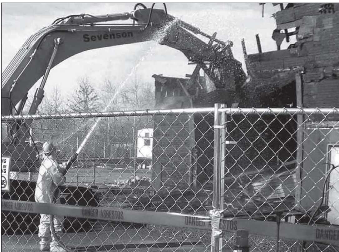
Demolition began at the Cornell-Dubilier Electronics Superfund site in February 2007.
