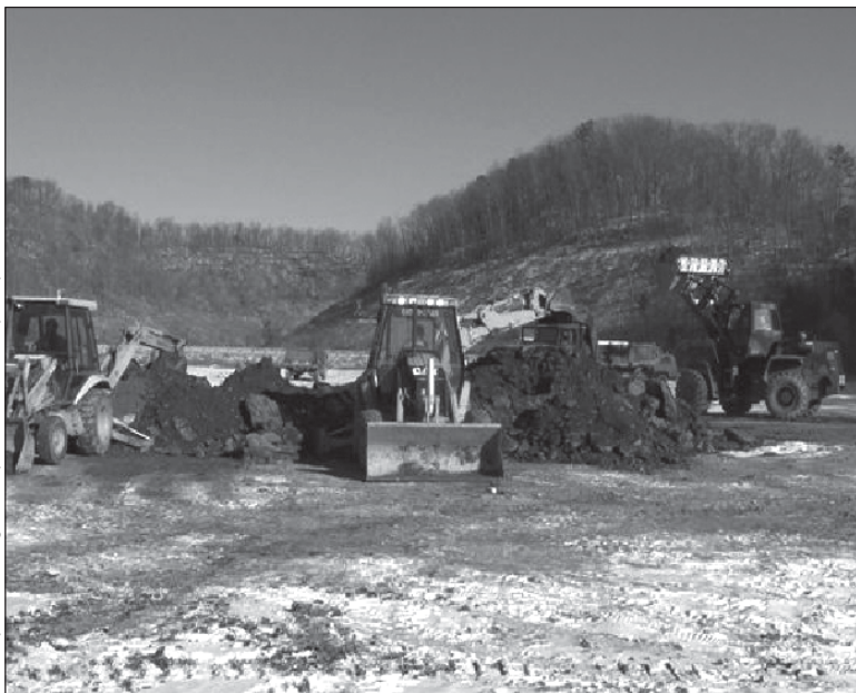
Soldiers from the 207th Horizontal Company, 201st Engineer Battalion, learn to operate loaders and backhoes.
