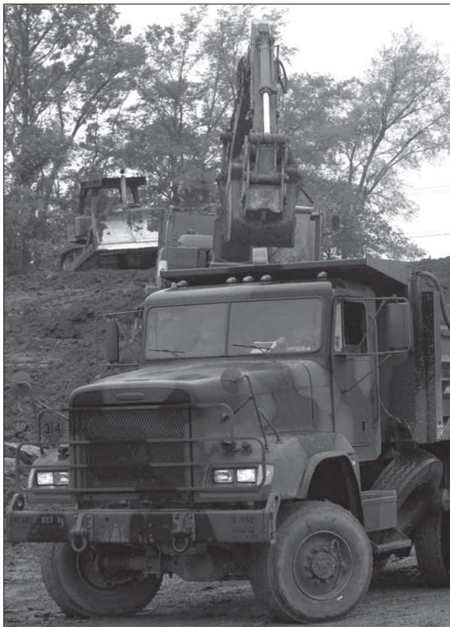
A hydraulic excavator fills one of the six 20-ton dump trucks on the project.
