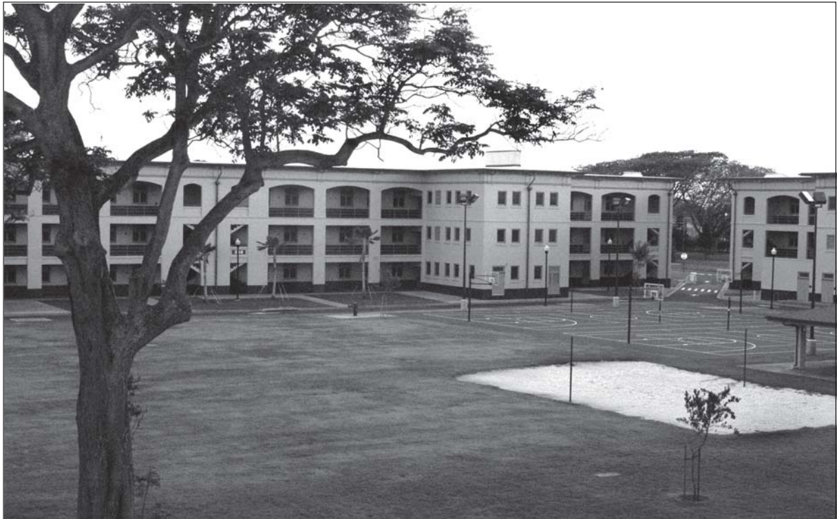
Newly renovated C Quad and courtyard
