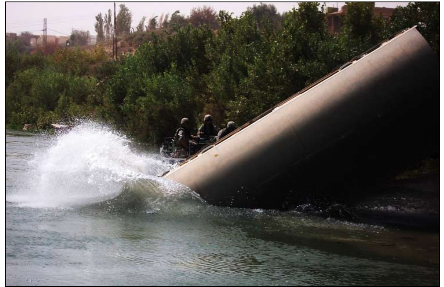
Soldiers of the 401st Multi-Role Bridge Company launch an interior bay into the Tigris River during a bridging project in Iraq.
