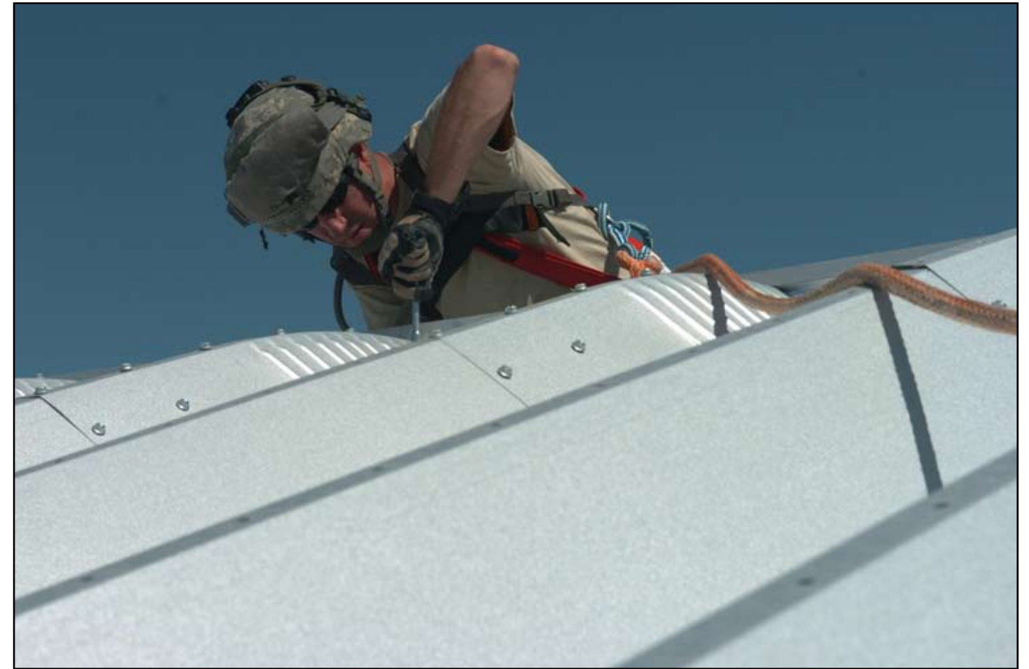
Sgt. Andrew Stang, a carpenter from the 492nd Combat Engineer Company uses a cordless drill to tighten bolts on top of a Quonset hut at FOB Miami during Operation Sand Castle 2009.
