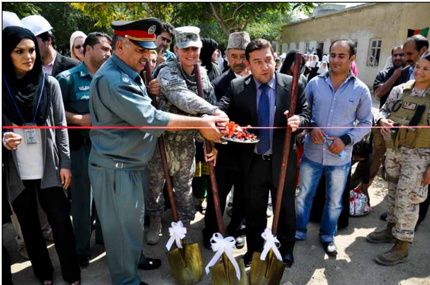
Representatives from NATO Training Mission - Afghanistan and the Ministry of Education cut the ribbon together on the construction site at the Bibi Hawa Elementary School Sept 7, 2011. They also took turns shoveling concrete into the spot where the cornerstone would go. Then they placed decorative stones signifying the first bricks of construction.
