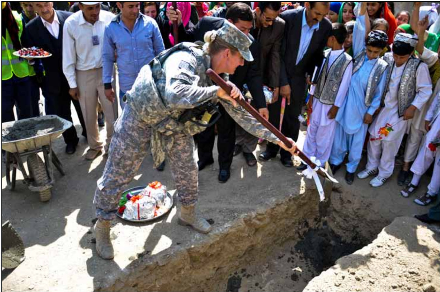
Army Col. Karen Saunders, Combined Security Transition Command - Afghanistan, shovels cement into a hole that signifies the beginning of a new school building. The Bibi Hawa Elementary School held a groundbreaking ceremony for their new building Sept. 7, 2011.
