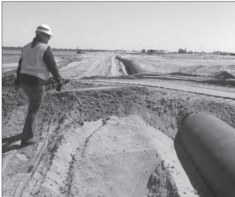
The team removed mounds of earth and vegetation from low-lying areas of the marsh.
