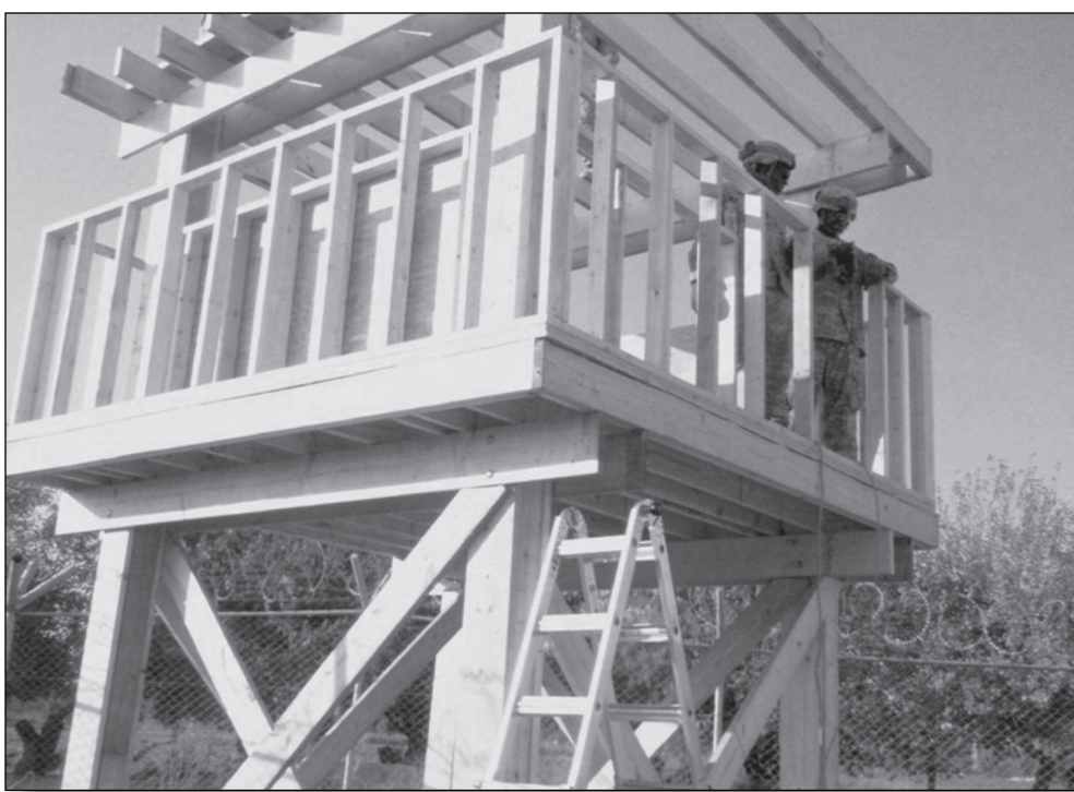
Standard Guard Tower Construction
