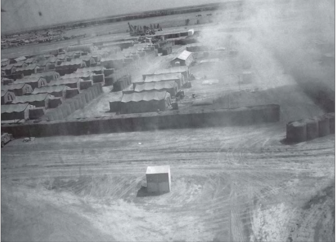
Construction of an engineer living area was a top priority.
