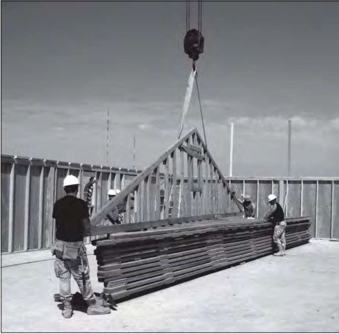
Airmen construct new headquarters facilities for brigade combat teams.
