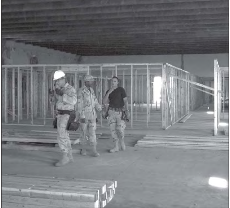
Airmen construct future brigade headquarters.
