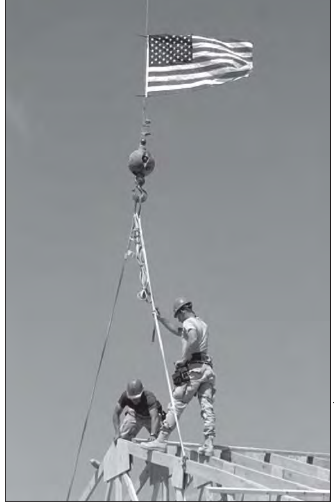
RED HORSE engineers install roof trusses as they build up FOB Hammer for the 3d BCT in Besmaya, Iraq.
