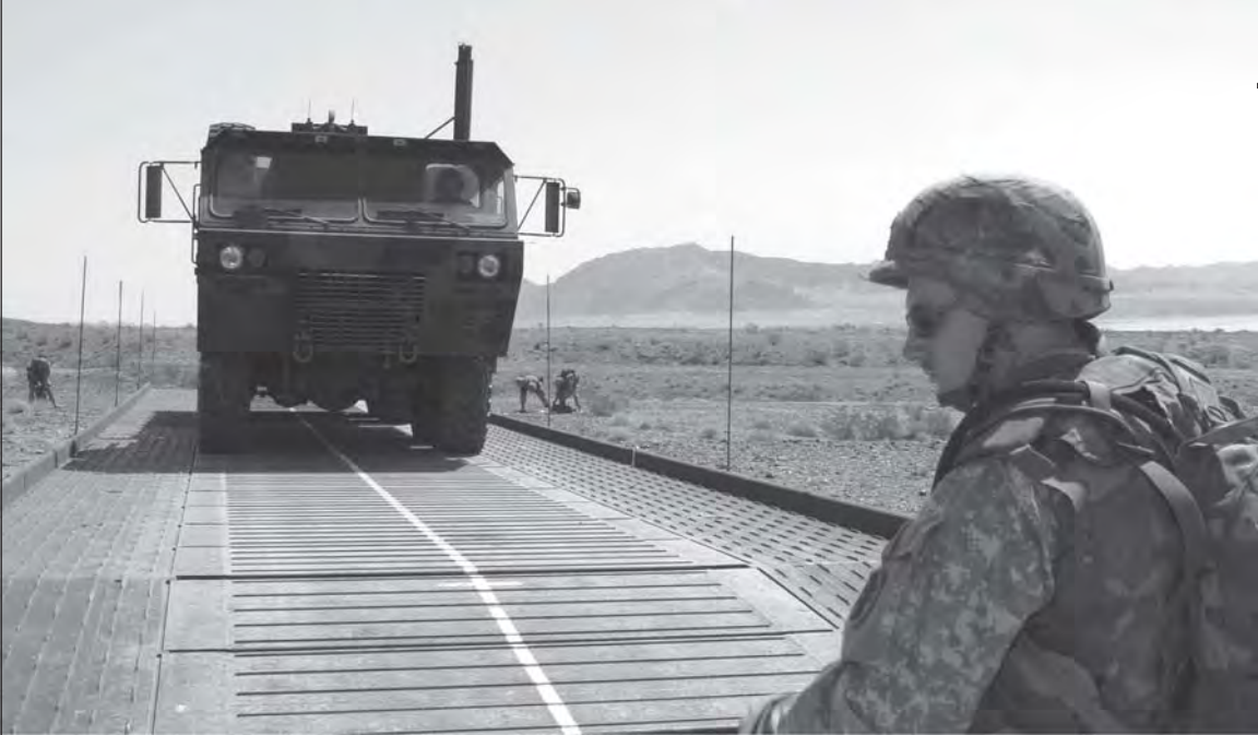
A 459th Engineer Company Soldier leads a truck across the dry support bridge that the company just set up.
