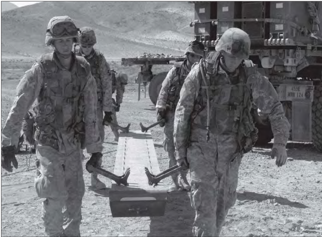
Members of the bridge crew with the 671st Engineer Company begin the breaking-down process of their dry support bridge after it was tested with tactical traffic.
