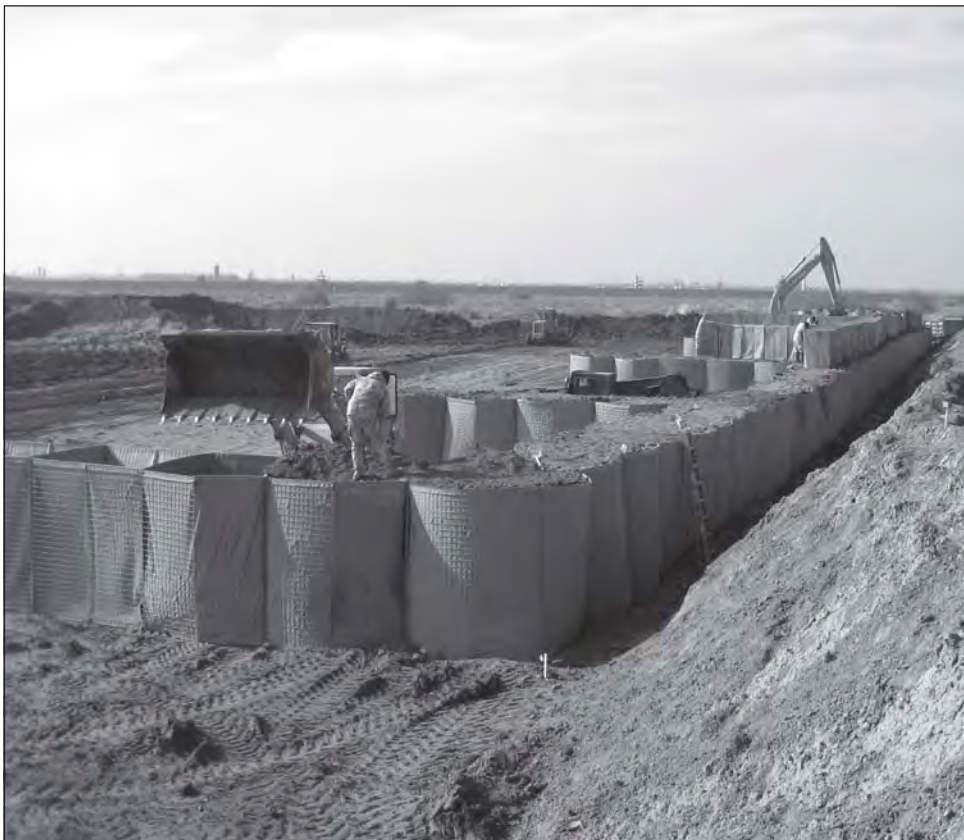
HESCO Bastion Concertainer® units surround an ammunition holding area.
