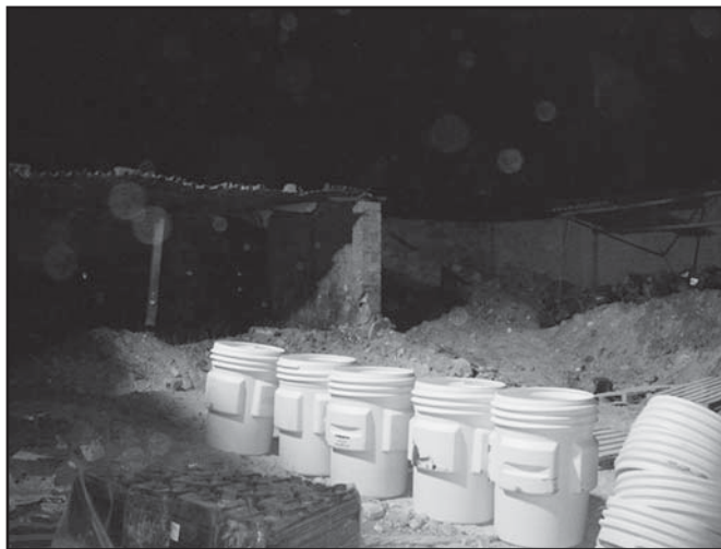
Overpack containers ready to be filled
