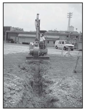
A Solutions-IES employee excavates a trench for the installation of a custom-engineered, belowgrade EOS recirculation system.
