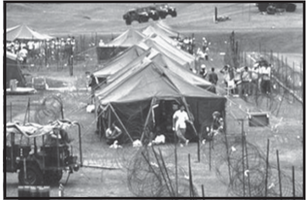
Partial view of the inprocessing area at the CDCC
