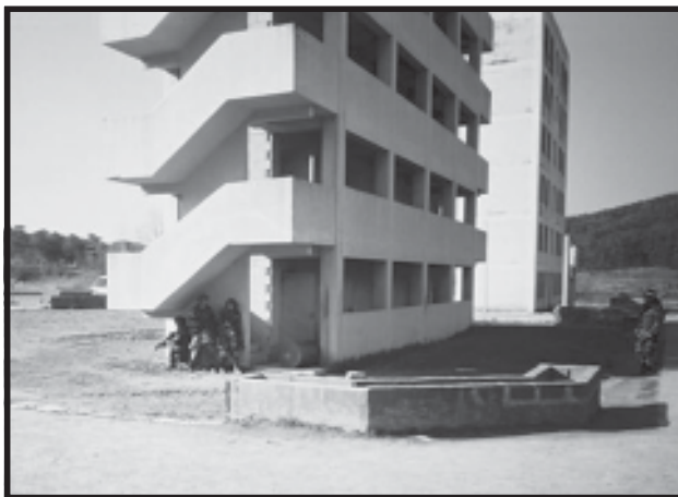
A team of three soldiers “stacks” on the door of a building at the Yongtari MOUT facility.
