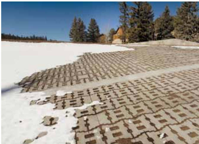
At top: Grace Lake Dam looking North. Above: Grace Lake Dam, articulated concrete mat blocks. Right: Leo Lake Dam demo. All photos by Harry Weddington
