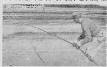
RE-SETTERS - These two have the job of resetting the cable once the aircraft lands. With split-second timing they can maneuver it back onto its supports and be ready for the next landing aircraft within minutes.
