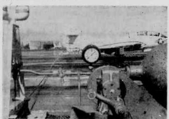
PRESSURE SET . . . GOOD CATCH — With a landing F9F in the runway. He then signals crew to background, this birds-eye-view of the arresting gear shows the recover cable and prepare for the pressure gauge which is one of the "keys" to the entire operation. next aircraft.
