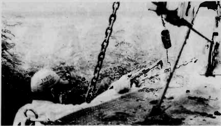
DISMANTLING HISTORY — Skip Ronning, a worker from the Metal Shop of the Facilities Department, begins to take apart the Ulupau Crater cable car. The cable car saw service from 1942 until 1970, transporting personnel 683 feet to the top of the Crater. (Photo by Sgt Chris Taylor)
