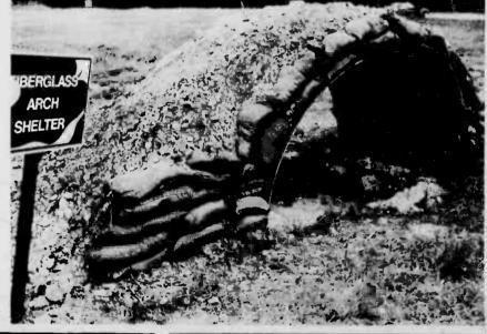
HOME SWEET HOME? - This protective shelter is being developed with the tank-killing TOW (tube-launched, optically-tracked, wire-guided missile) in mind. The shelter, plus 18 inches of dirt, allow the guile growt. allow the gun's crew to retaliate against enemy armor during bombardment. (Photo by Sgt Christopher Grey)
