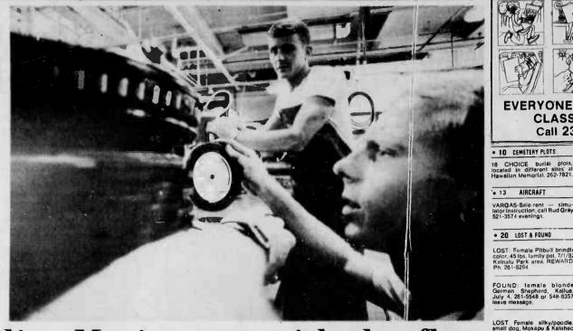
UNDER PRESSURE - Sergeant Rick Schmidt watches the pressure gauge, as Lance Corporal Ronald Mills, applies pneumatic pressure to an F-4S Phantom brake. Both Marines are hydraulics mechanics at Headquarters and Maintenance Squadron-24's Hydraulics Shop. (Photo
