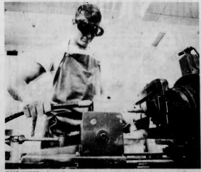
HOSE MAKER - Lance Corporal Ronald Mills, hydraulics mechanic, manufactures an hydraulic hose using the hose assembly
