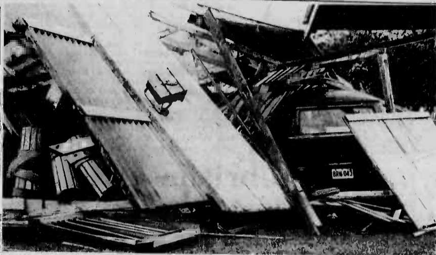
THE BUILDING THAT WAS — A Volkswagen bus lies buried beneath rubble that was once part of the Station Fire Department. (Photo by Sgt Chris Taylor)
