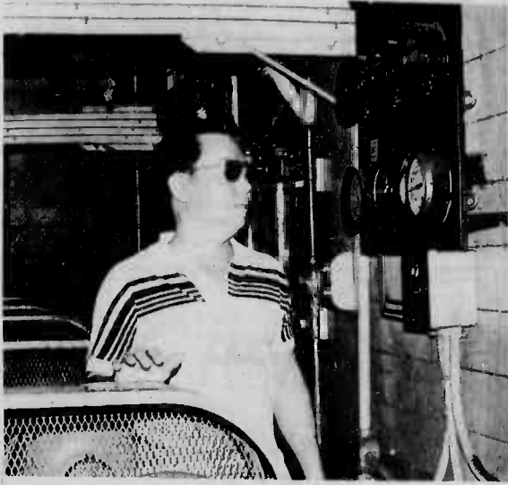
BENEFICIAL SUGGESTION WINNER — Steven Fujiyoshi, shop planner of Facilities Department here, checks the pressure rating of suction and discharge gages inside a refrigeration system compression room.
