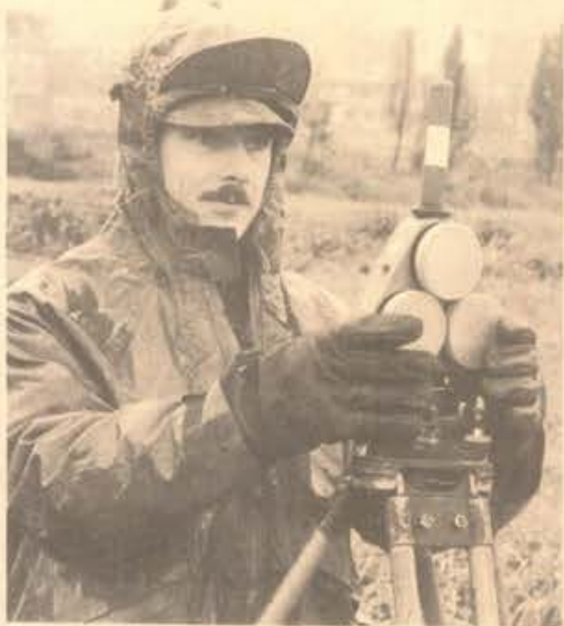
DEADEYE — A Marine from the TOPO surveying team assigned to the 24th Marine Amphibious Unit demonstrates the use of the Theodolite T-2000 surveying instrument.
