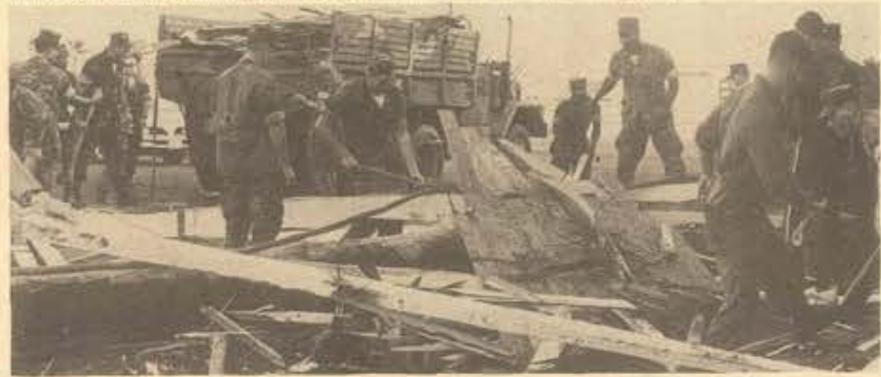
HURRICANE DAMAGE — Workers clear rubble left by the passing of Hurricane Iwa. The 1982 hurricane unleashed 130 mph winds causing millions of dollars worth of damage just before Thanksgiving.
