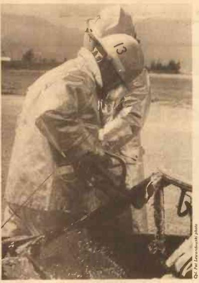
Sergeant Mark Hilts, a Crash, Fire and Rescue firefighter, cuts through a roof support using large pneumatic crimpers, while Staff Sergeant Demont Macklin backs him up. Abandoned vehicles are used by Marines to practice forced
