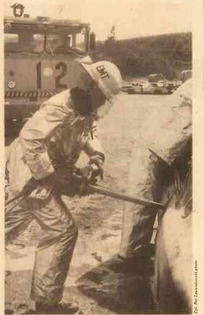
Staff Sergeant Demont Macklin Station Operations and Maintenance Squadron, Crash, Fire and Rescue section leader, uses pneumatic "jaws" to open the door of a wrecked vehicle. Using abandoned cars to simulate aircraft cockpits, the Marines from CFR can practice life-saving techniques otherwise only covered in the classroom.
