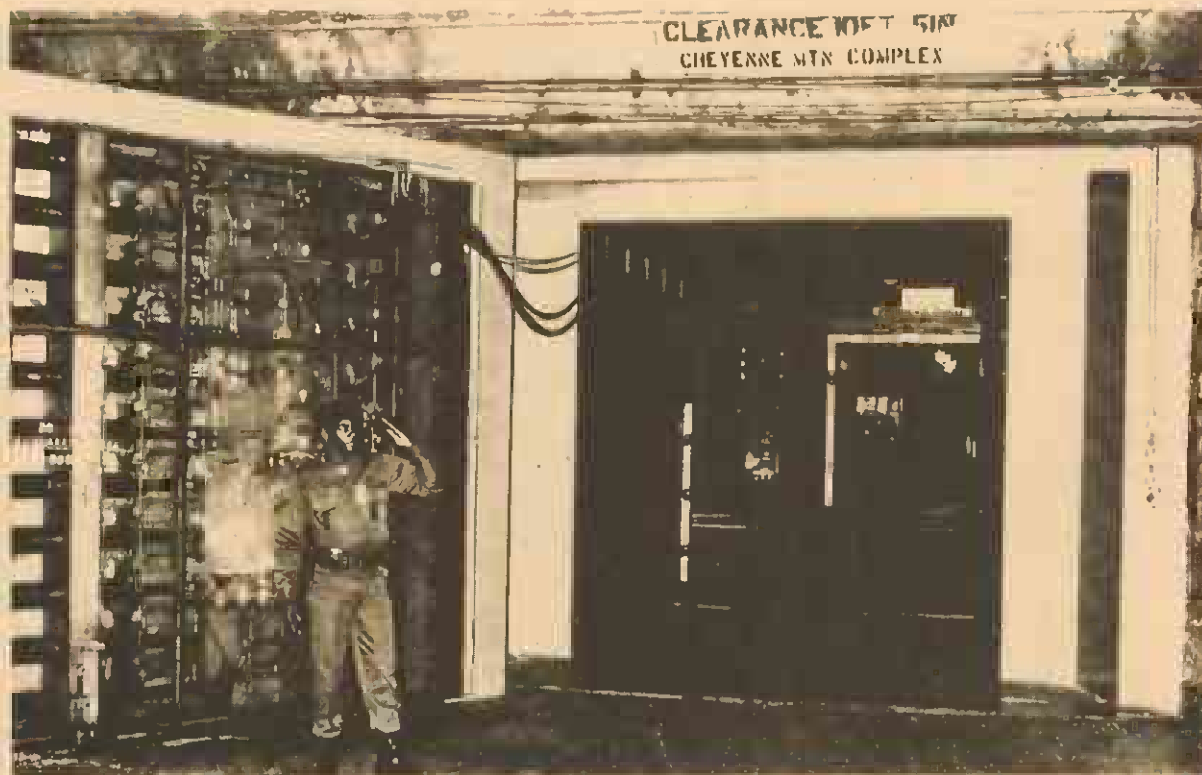
Massive blast doors, more than three feet thick and with a swing weight of 25 tons each, protect the entrance to the Cheyenne Mountain complex. Hydraulically operated, they can be opened or closed in 45 seconds.
