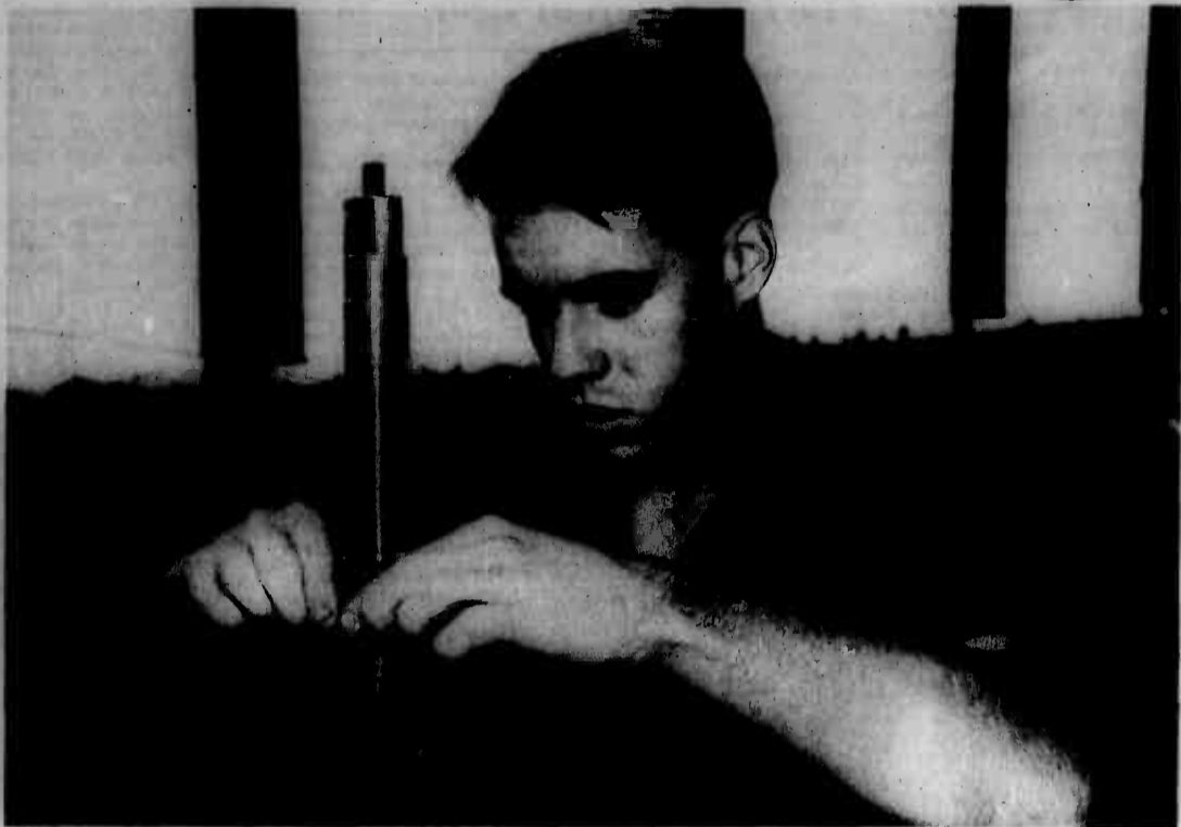
Lance Corporal Cliff C. Clowers, an engine mechanic at H&MS-24, replaces a bearing on a power turbine rotor.
