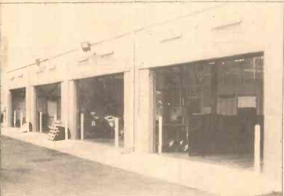
With 15 indoor bays, the new Auto Hobby Shop also provides a variety of services and improvements.
