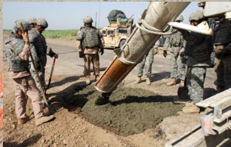
Left: Spc. Brad Buehler maneuvers a nimble bobcat with a jackhammer attachment to even out the edges of a blast hole. Below left: Spc. Chris Fitzsimmons uses skills learned as a civilian equipment operator to deftly manipulate a backhoe. Below: Cement is poured into the former blast crater. Bottom: Sgt. Jason Bolin puts some muscle into smoothing a patch of concrete poured over a blast hole on Route Heather. Once the patch is dry insurgents will have one less place to hide IEDs.
