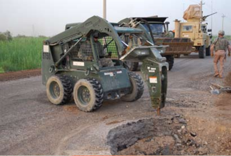
Left: Spc. Brad Buehler maneuvers a nimble bobcat with a jackhammer attachment to even out the edges of a blast hole. Below left: Spc. Chris Fitzsimmons uses skills learned as a civilian equipment operator to deftly manipulate a backhoe. Below: Cement is poured into the former blast crater. Bottom: Sgt. Jason Bolin puts some muscle into smoothing a patch of concrete poured over a blast hole on Route Heather. Once the patch is dry insurgents will have one less place to hide IEDs.
