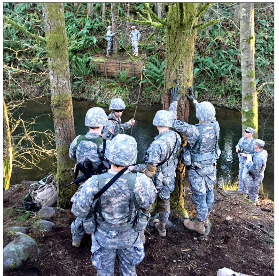
Members of the University of Alaska ROTC Ranger team construct a rope bridge during the 8th Brigade Ranger Challenge Finalists Competition at Joint Base Lewis-McChord, Feb. 27 and 28. (Courtesy photo)
