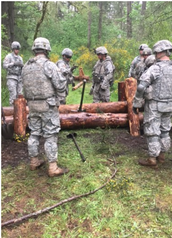
2nd PLT emplaces a Log Crib during the VALDEX in May 2015
