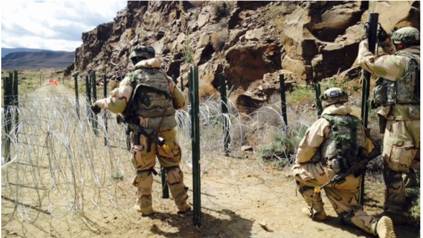
3rd PLT emplaces an 11-Row wire obstacle while support 1-23IN at Yakima in April 2015
