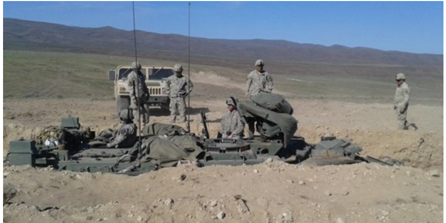
Stryker Turret Defilade Fighting Position dug by the EQ Platoon at YTC Rotation
