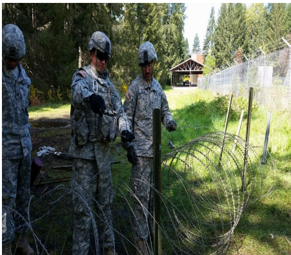
3rd Platoon “WolfPack” work on counter-mobility tasks by emplacing wire obstacles.
