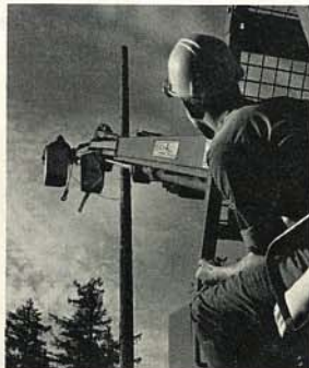
AIR GUARD COMMO experts reach skyward while building "antenna farm."
