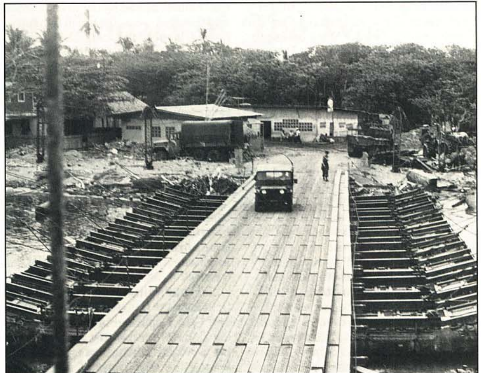
Training in Panama, Tennessee Guardsmen test newly-erected floating bridge that spans watery trade barrier for natives.
