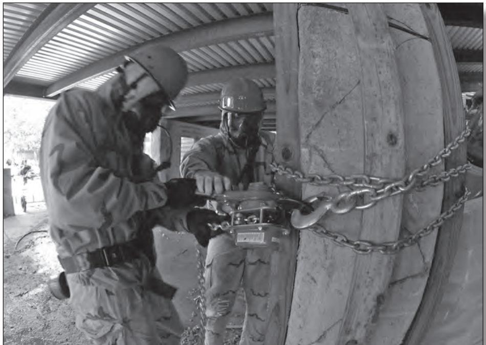
Engineers from the 178th Engineer Company apply wooden bracing and linked chains to a pillar supporting a collapsed parking garage during a field training exercise.
