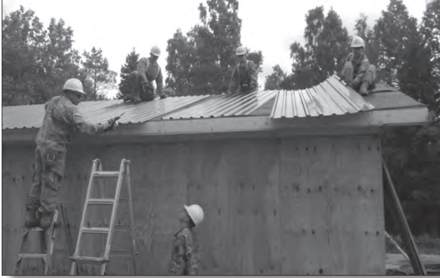
U.S. Soldiers build a multipurpose range facility in Tapa, Estonia.
