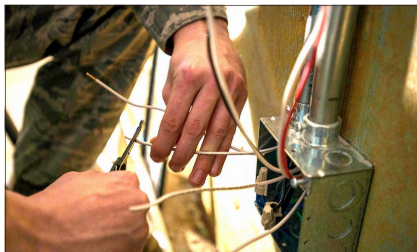
Airman 1st Class Sprinkles is shadowed by work lights while he roughs in wires during a remodel in Amber Hall on March 3, at Eielson Air Force Base, Alaska. With the lights off deep in the basement, the wiring is the ground work that will power office space to support missions across the U.S. Pacific.
