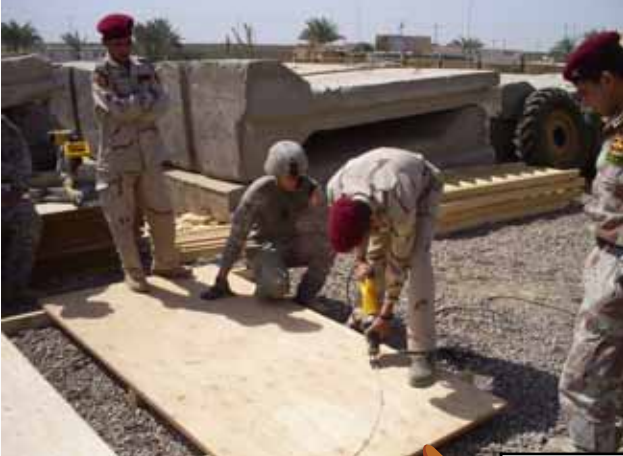
Sgt. Mark Jordan, instructs a team of 23rd Iraqi Army Engineer Regiment Soldiers on how to outfit their concrete guard towers with wooden safety platforms.
