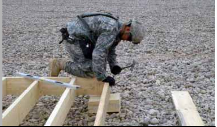
Spc. Chance Bailey from Russellville, Ark, nails together a floor system frame to prepare it for sheathing. The 46th Eng. Bn. is building 30 B-Huts, a dining facility extension and a food preparation area at Combat Outpost Carver, located in the southeastern outskirts of Baghdad, May 4.
