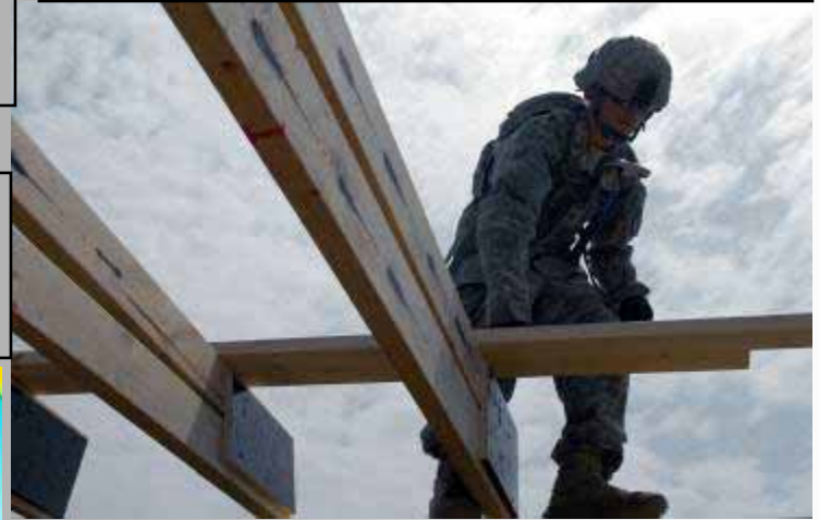
Spc. Chance Bailey from Russellville, Ark, nails together a floor system frame to prepare it for sheathing. The 46th Eng. Bn. is building 30 B-Huts, a dining facility extension and a food preparation area at Combat Outpost Carver, located in the southeastern outskirts of Baghdad, May 4.
