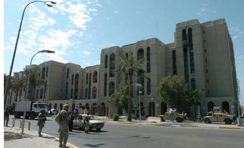
Soldiers with Special Troops Battalion, 2nd Brigade, 1st Cavalry Division's Infrastructure Coordination Element walk down Haifa Street in Baghdad's Karkh District to assess damage caused by fighting there.
