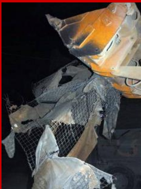
Hesco barrier removal along Abu Nuwas Street was further proof of the implementation of the Security Agreement as Combat Outpost 102 in the Rusafa district of Baghdad, May 28. The engineers from the 46th Engineer Combat Battalion (Heavy), 225th Engineer Brigade performed the nighttime mission at the direction of the 3rd Brigade Combat Team, 82nd Airborne Division.
