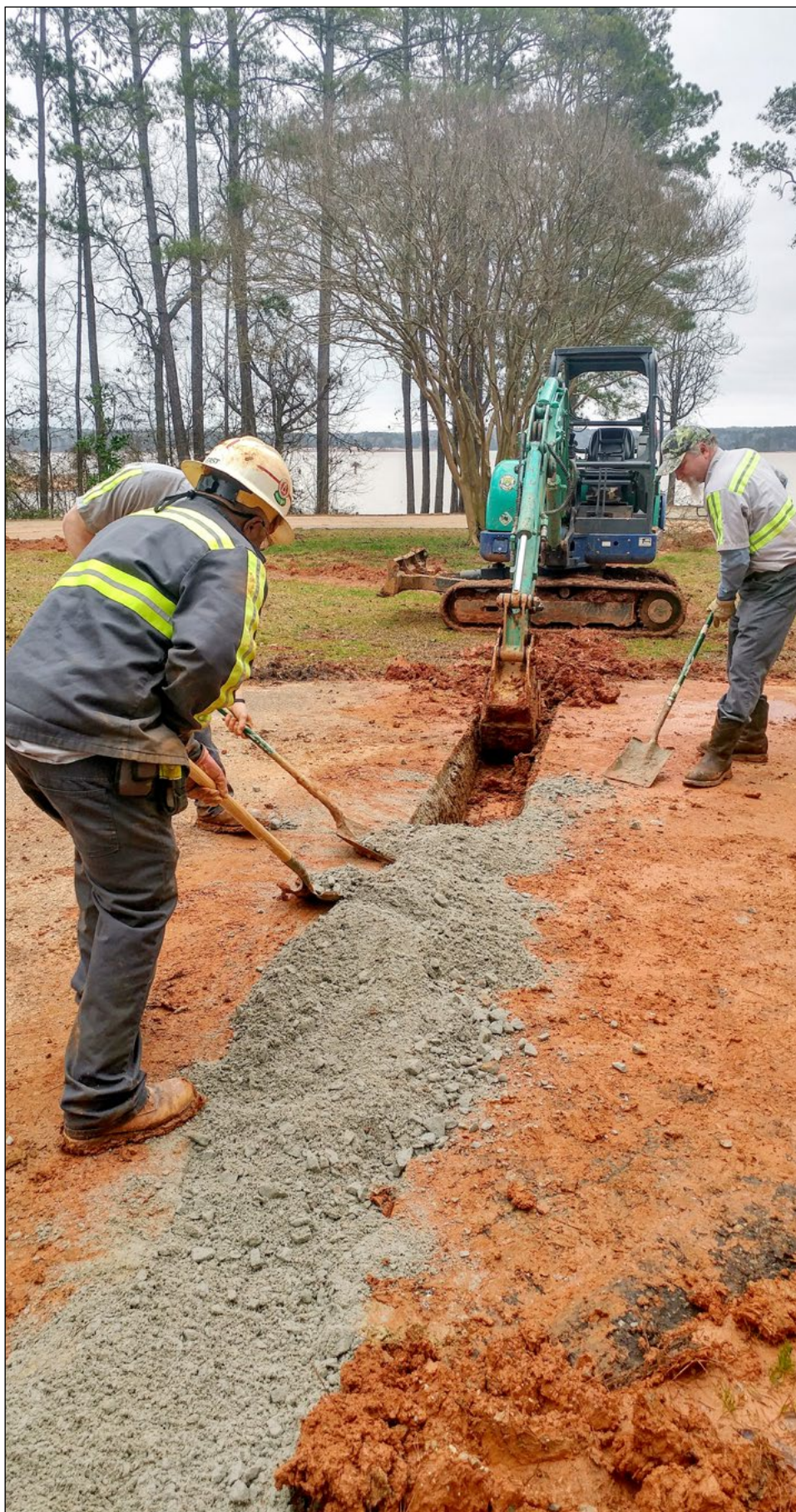
Contractors install a new water line at Whitetail Ridge Campground on the western shore of West Point Lake along the Alabama-Georgia state line. (Photo courtesy of West Point Project)
