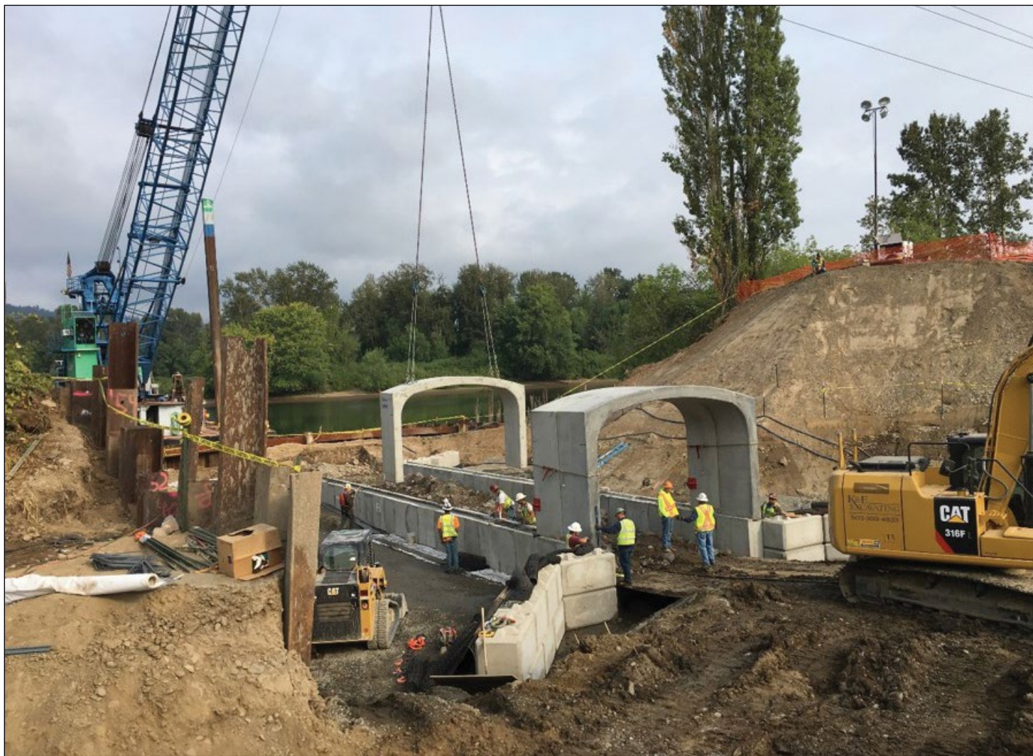
A crane lifts one of the culvert sections into place. The precast culvert pieces were formed off-site and brought in by barge to allow for faster assembly and to decrease the project's footprint.
