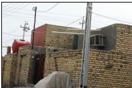
Turning up the power, p. 6
